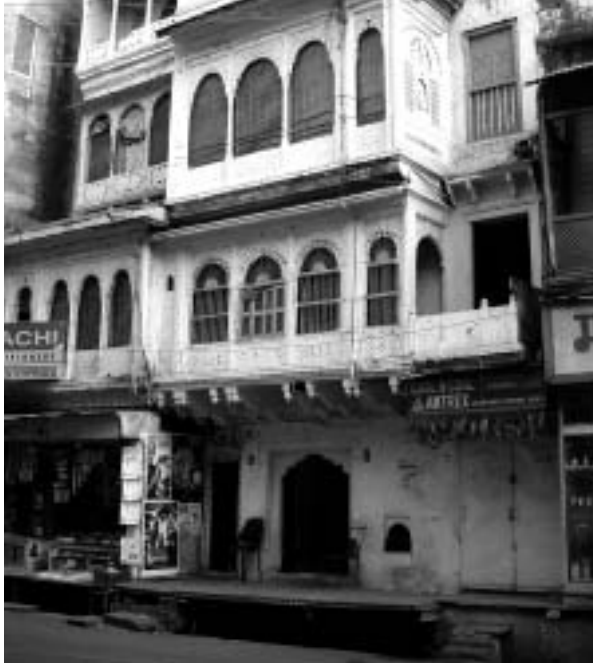
Singhi House- a typical house in the commercial cum residential street, shop at ground floor, residence at upper floors, first floor projected on stone brackets, recessing upper floors with perforated fascia.
