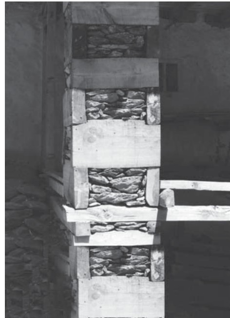
Thathara - A typical wood-n-rubble pillar
