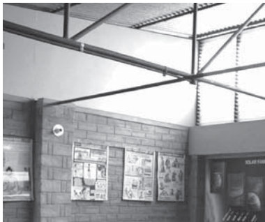
Flyash and waste residue wall
