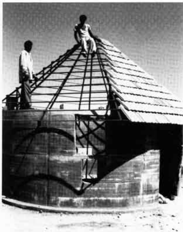
Rammed earth circular structures, Source: Hunnarshaala
