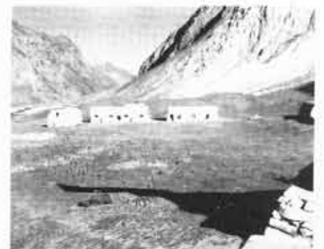
PANCHTARNI NIGHT HALT POINT EXISTING PERMANENT SHELTERS
