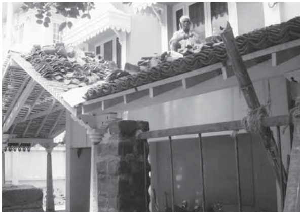
Skilled local labour and artisans are regularly employed by the INDeco Hotels. Seen here is a locally employed roofer laying tiles on a roof
