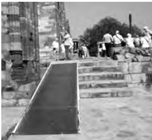
Before audit-inaccessible ramp at Iron pillar
