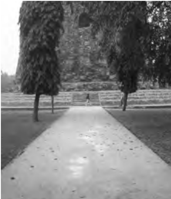
Accessible pathway has been created at Qutb Minar by levelling the surface and removing the gravel for the benefit of visitors with reduced mobility
