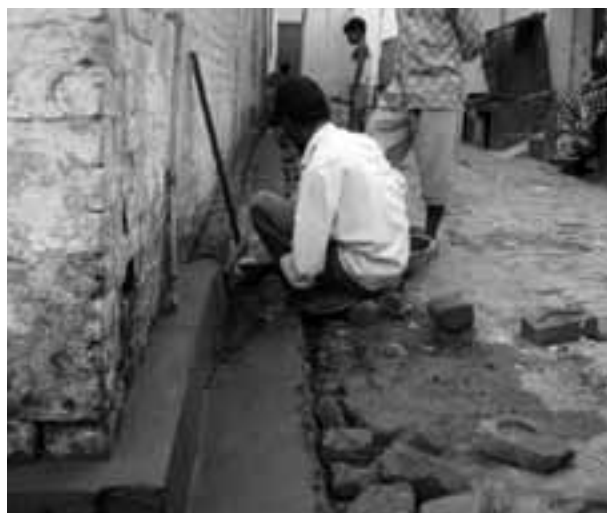
Constructing drains
