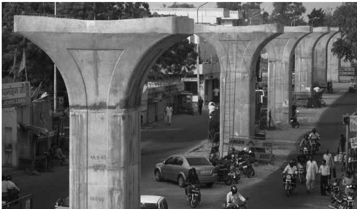
Elevated road for Bus Rapid Transit System under construction, Jaipur
