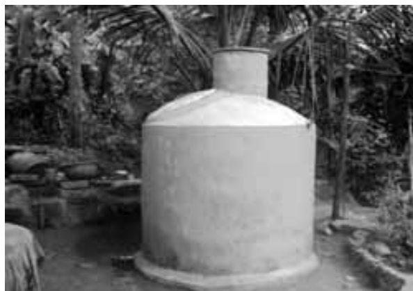
Construction of bio-gas digester in progress
