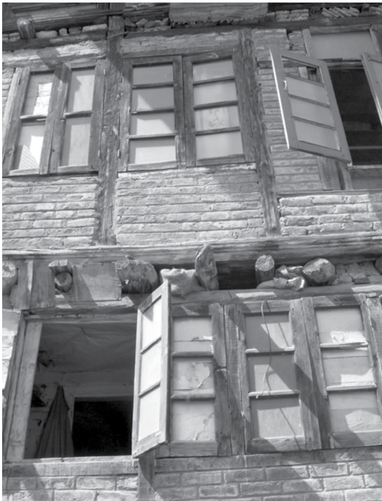
Tradition timber framed construction in Dhajji Dewari. This is one of the safest construction methods for buildings to withstand earthquakes in Srinagar, Kashmir
