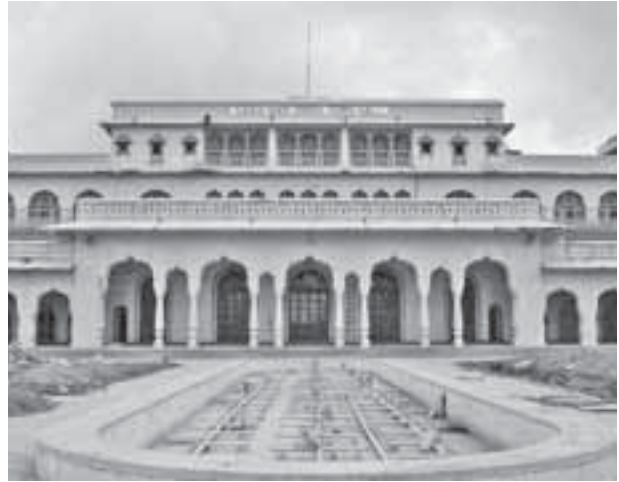
Front elevation of the Old Vidhan Sabha designed by Samuel Swinton Jacob
