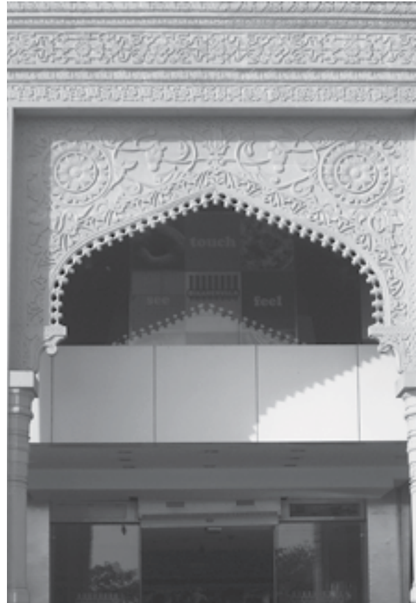
An arch clad over a modern steel and glass facade in Gurgaon
