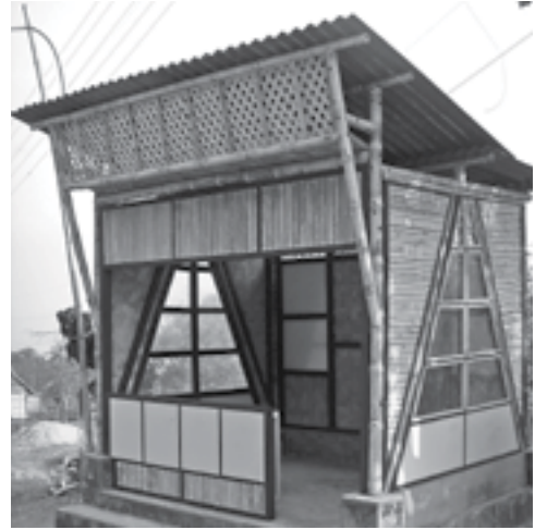
Bamboo structure exploring innovative and alternative use of Bamboo. Source: NBDA
