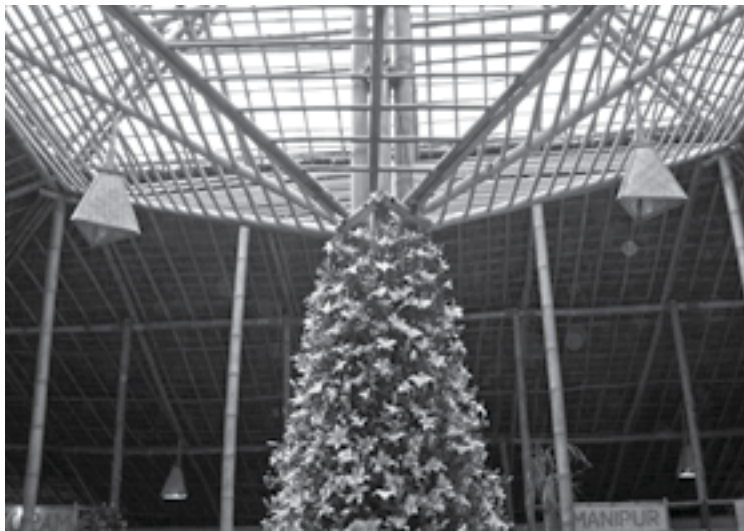
Bamboo structure at Naga Heritage Village. Source: NBDA
