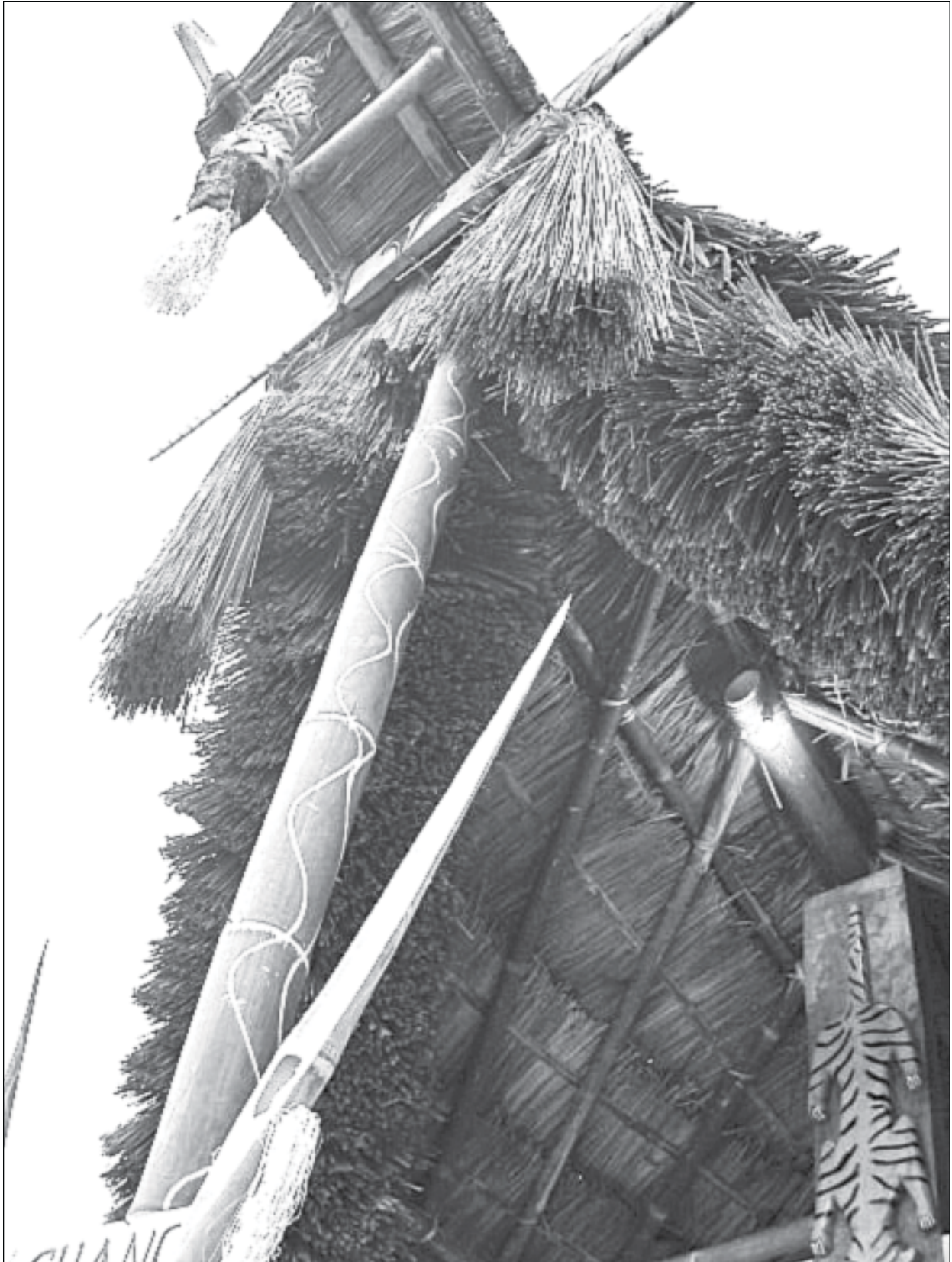
Typical, heavy overhanging roof made of palm thatch
