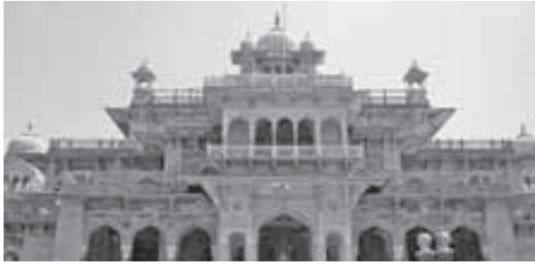
Front view of Albert Hall, Jaipur
