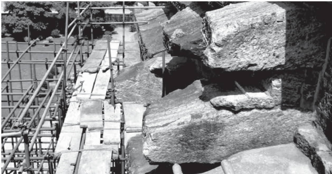
Loose stones on the left facade of Jagamohana roof. Source: Photograph by Author for ASI
